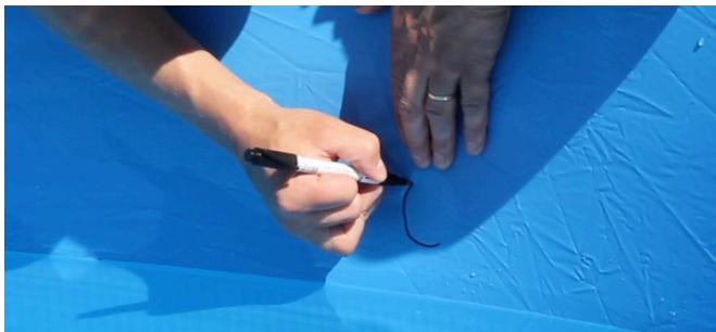
Draw/mark the round hole in the liner and then cut an X in the circle with a sharp knife. Do not cut beyond the marked hole. Now fit the return tube (11) and a gasket (12) from the inside of the pool and out through the pool wall. Attach the return tube to the pool wall by firmly tightening the plastic nut (13). Do not overly tighten the nut. Odt fast. Undgå at overspænde omløberen.
