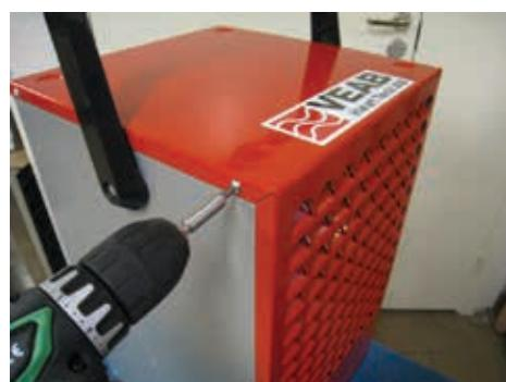
When cleaning is needed loosen the upper casing.
