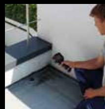
Discover leaks in roofs
