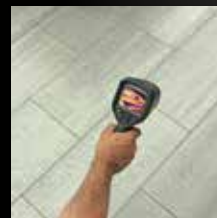
Check floorheating for leaks
