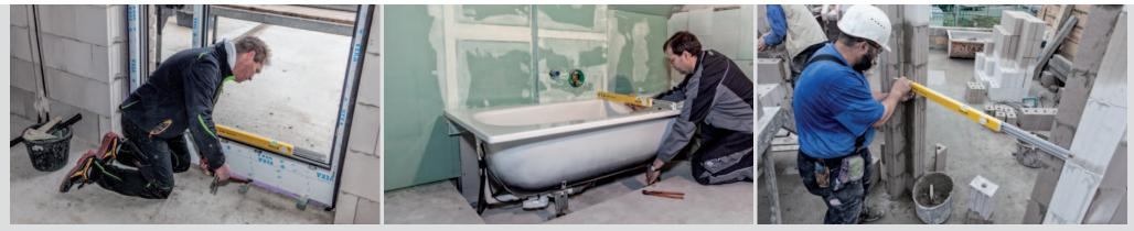
Thanks to the telescopic system, the tradesman can set the spirit level to precisely the length needed for the job.
